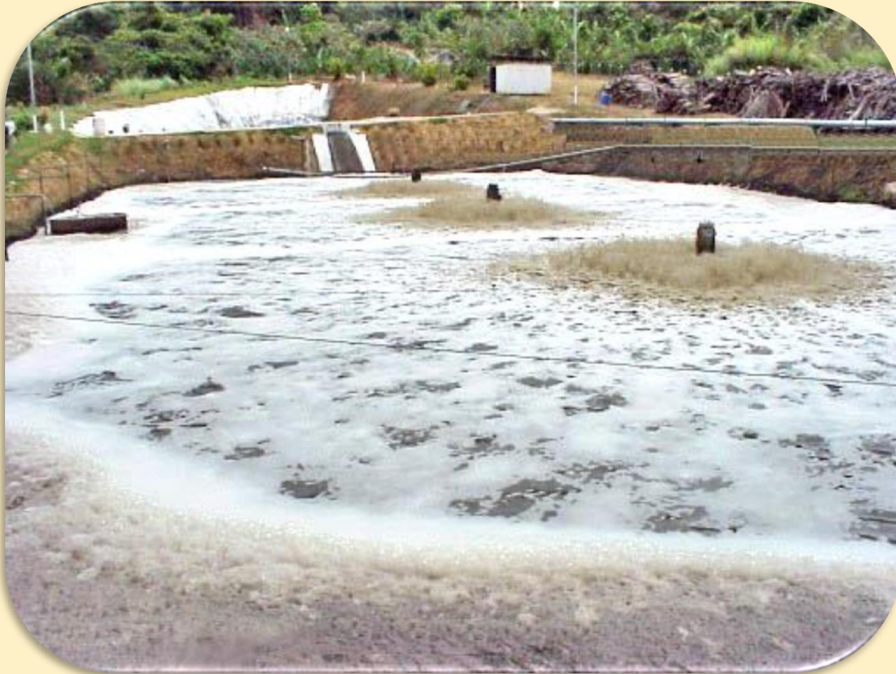
Oxygenation pond with aerators Precipitation of solids
